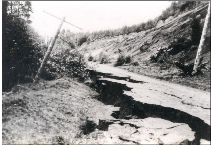
Figure 2 Chasm in Kelsey Bay highway, just north of Campbell River
